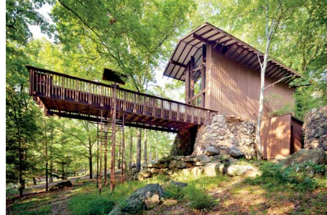
Fay Jones's hit upon his magical 2:4:5 formula for proportions in the dimensions of Stoneflower, which is twelve feet wide, twenty-four feet tall, and sixty feet long, including the deck.
